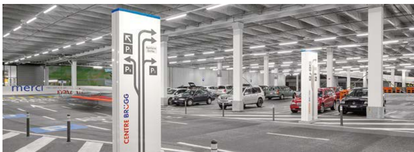
Light lines arranged along both sides of the driveways serve as visual crash barriers.
