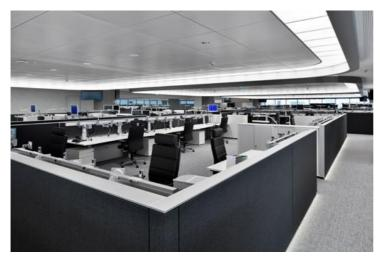
**Photo 2:** The customised lighting solution by Zumtobel uses illuminated ceiling panels made up of backlit micro prismatic panels to obtain a skylight effect and to convey an impression of daylight for workplaces that are situated well away from any windows.
