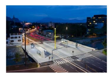
**Photo 3:** The key challenge for the lighting solution was to ensure a uniform illumination that covered the total area and complied fully with the relevant standards for road transport, cycle paths and pedestrian crossings.
