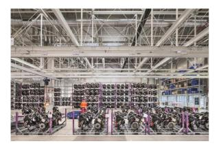
**Photo 2:** A total of 16,000 TECTON luminaires are installed in the factory on trunking that covers a distance of around 40 kilometres.
