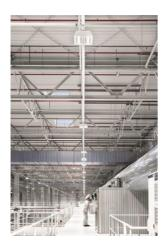
Photo 3: The CRAFT L high-bay solution is installed in the paint shop and higher halls.
