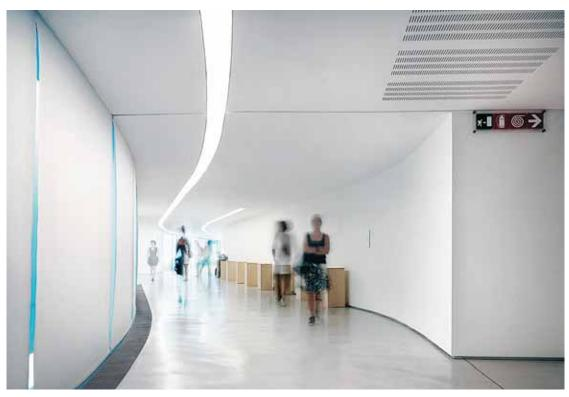
B5 I The lighting is integrated in the ceiling as a continuous light band and also provides an even illumination of the walls.
