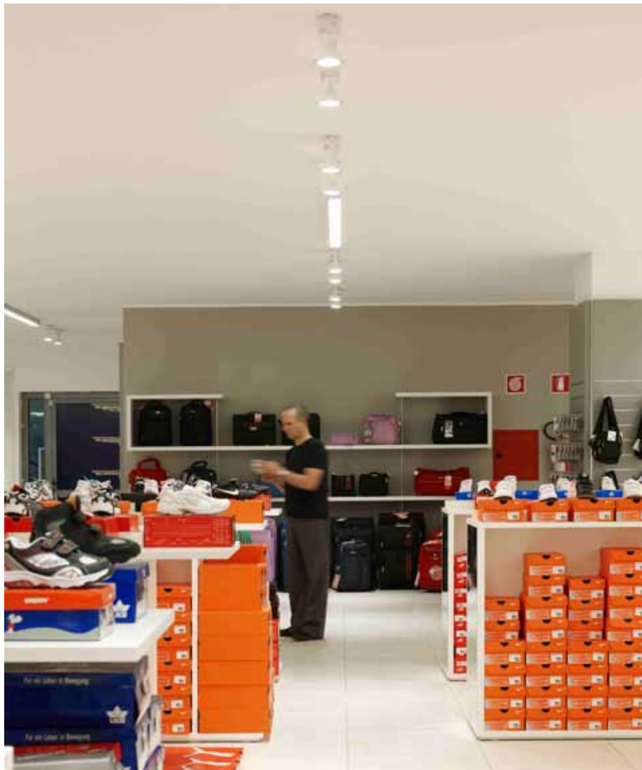
B2 | Slotlight light lines support the accent lighting provided by Discus spotlights with uniform ambient lighting.
