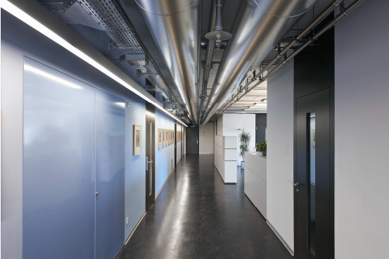
Caption 2: One of the two corridors remained unchanged, the other corridor was fitted with innovative Slotlight LED luminaires by Zumtobel
