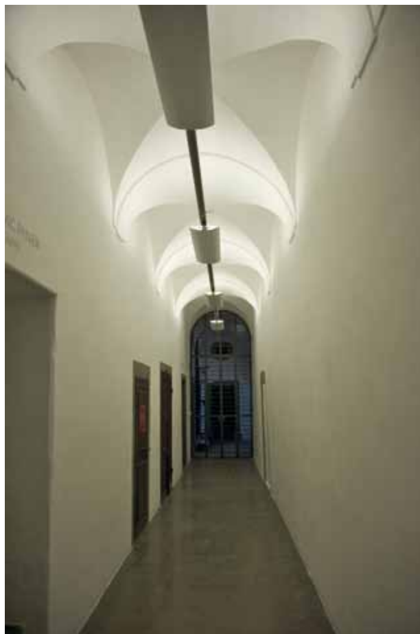
B2 | The historic cross vault is gently illuminated by the indirect light provided by the Tecton continuous-row lighting system.
