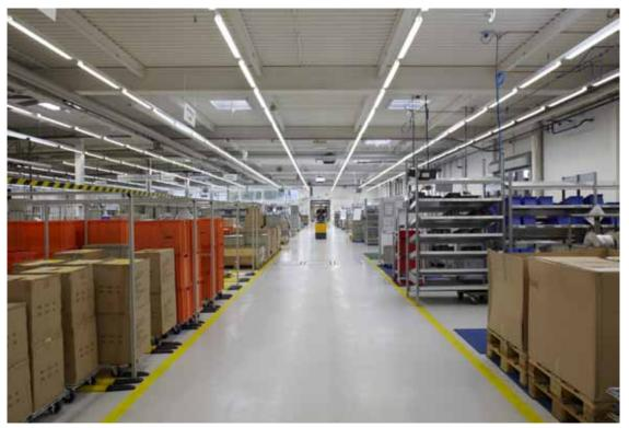
B2 I Improved lighting quality, less energy: the Tecton continous-row lighting systems are controlled via an intelligent lighting management system. In this way, just enough artificial lighting is added to provide the optimum illuminance level of 500 lux required. The daylight-based lighting system saves up to 50% of energy.
